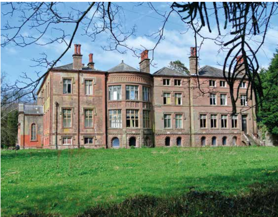
FIGURE 2.c.7.14 The late 18th (1780) century mansion at Calder Abbey, built on the remains of a monastery which had been established in 1142 AD
