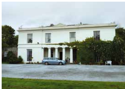
NO. 11 FIGURE 2.c.6.13 Steelfield Hall
