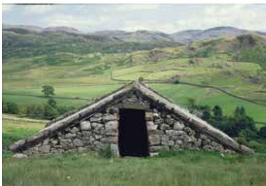
NO. 6 NO. 1 FIGURE 2.c.5.8 Peat huts above Boot, Eskdale
