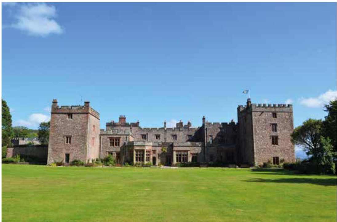
FIGURE 2.c.5.15 Muncaster Castle, a 14th century fortified tower overlooking the lower Esk valley, was extensively re-modelled in the 19th century
