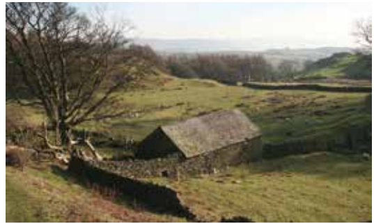
NO. 2 FIGURE 2.c.4.4 Stickle House Barn
