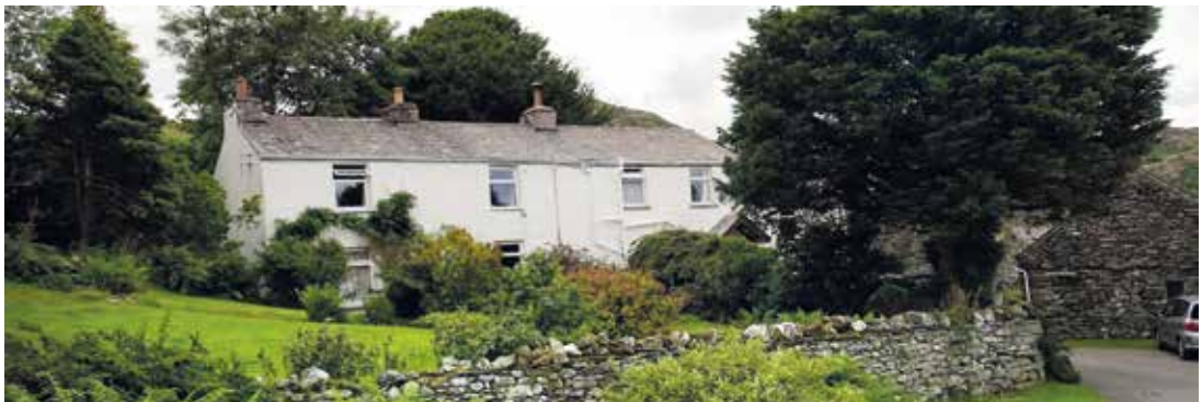
NO. 5 FIGURE 2.c.4.7 Stephenson Ground
