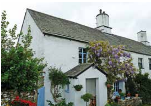
NO. 5 FIGURE 2.c.2.19 Plumgarths Cottages
