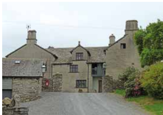
NO. 4 FIGURE 2.c.2.18 Hodge Hill Hall, Cartmel Fell
