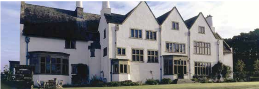
NO. 11 FIGURE 2.c.2.25 Blackwell (owned by Lakeland Arts)
