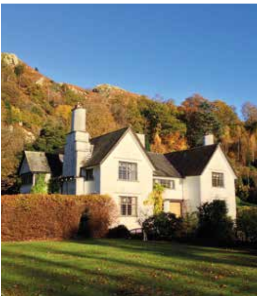
FIGURE 2.c.13.17 White Craggs, an Arts and Crafts style villa at Clappersgate at the head of Windermere
