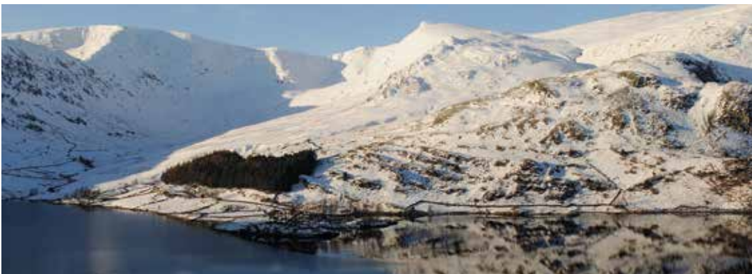
FIGURE 2.c.12.1 A view of the reservoir at Haweswater
