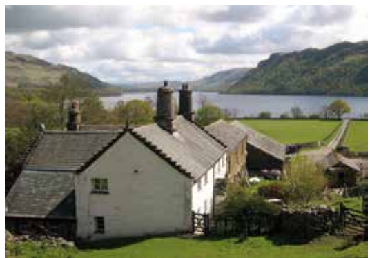
NO. 3 FIGURE 2.c.11.5 Glencoyne Farm (owned by National Trust)
