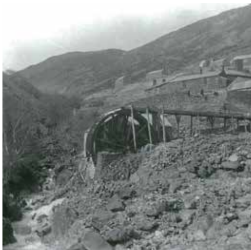
FIGURE 2.c.11.19 A view of a waterwheel at the Greenside lead mine (early 20th century)
