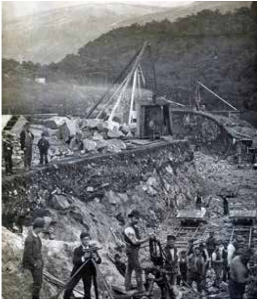
FIGURE 2.c.10.17 Thirlmere dam under construction, c. 1890
