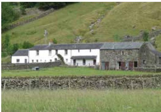
NO. 6 FIGURE 2.c.10.8 Fornside
