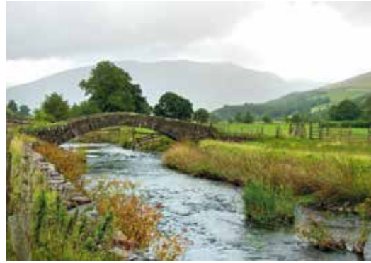
NO. 9 FIGURE 2.c.10.11 Sosgill packhorse bridge
