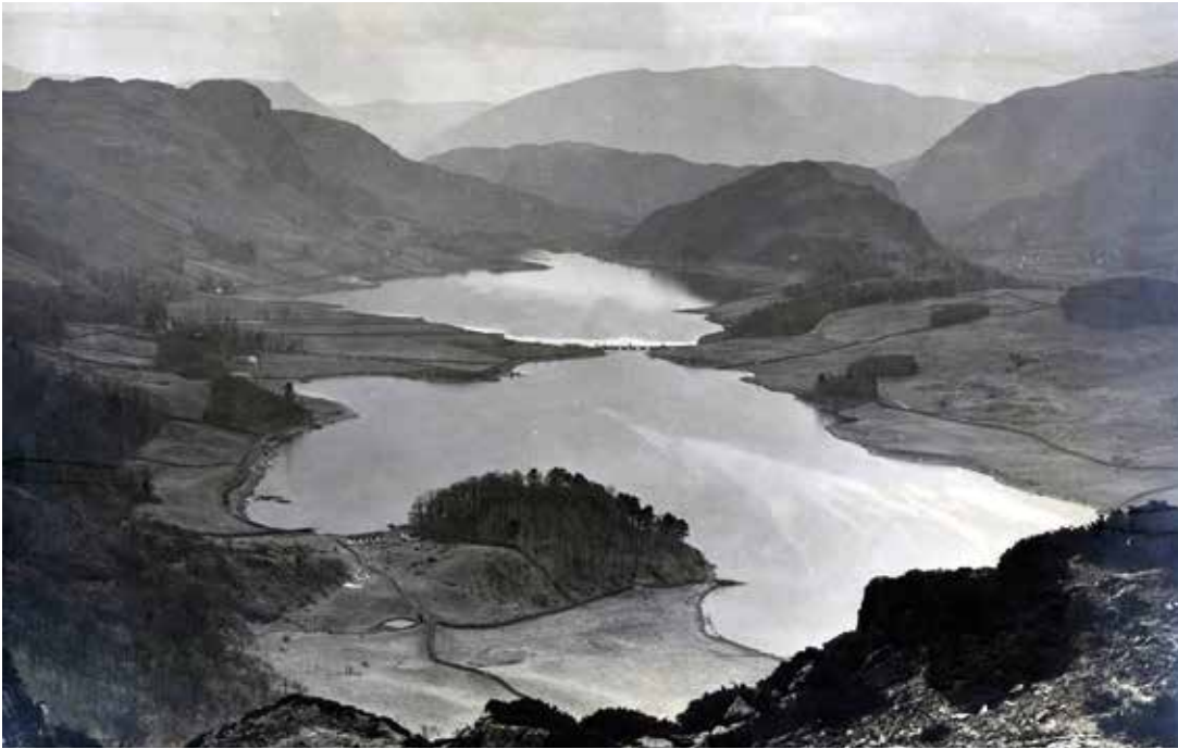
FIGURE 2.c.10.15 View north across Leathes Water prior to construction of the dam
