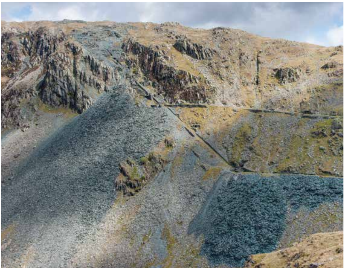
FIGURE 2.b.35 The slate quarries at Honister House, showing inclines, access tracks and waste heaps
