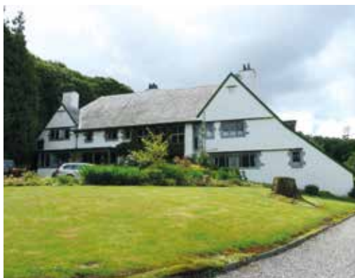
FIGURE 2.b.64 House in Arts and Crafts style at Moor Crag, Windermere
