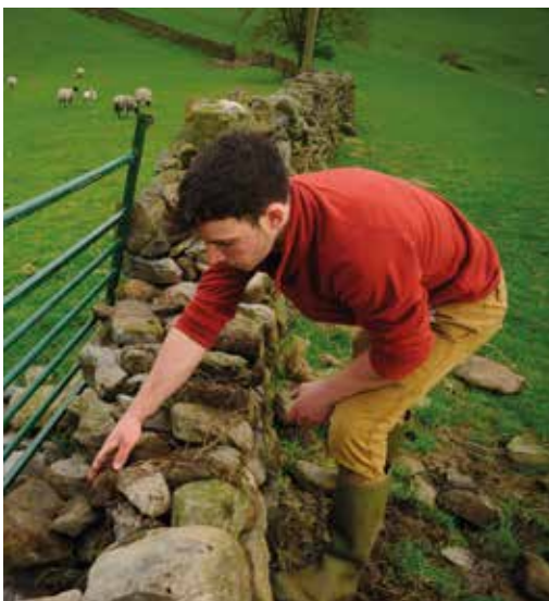
FIGURE 2.b.26 Repairing a stone wall
