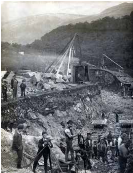
FIGURE 2.b.74 Thirlmere dam under construction
