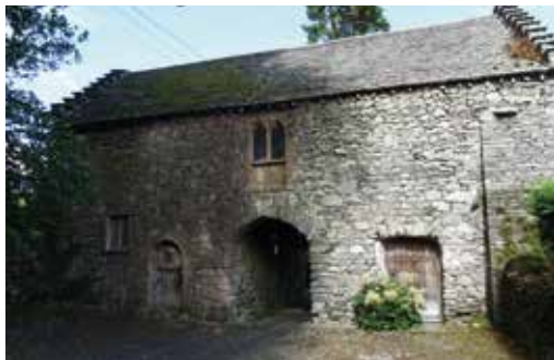
FIGURE 2.b.11 Hawkshead Courthouse, Coniston, associated with Furness Abbey's grange
