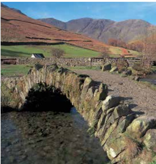
FIGURE 2.b.19 Row Bridge, Wasdale. A typical single span packhorse bridge
