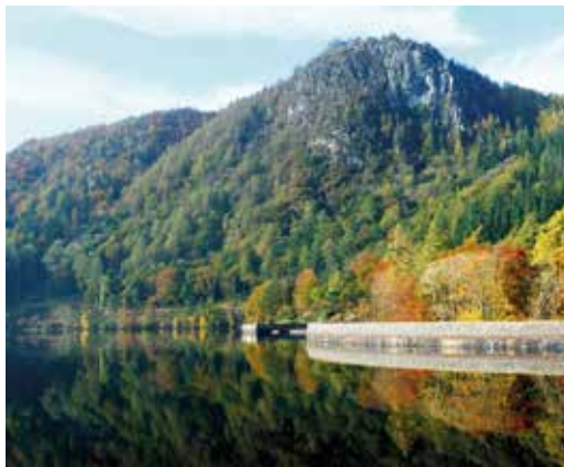
FIGURE 2.a.108 The dam at Thirlmere
