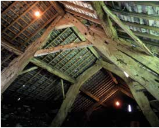
FIGURE 2.a.73 Re-used medieval wooden crucks in Fieldhead Barn, Outgate, near Hawkshead
