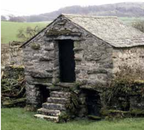
FIGURE 2.a.72 Piggery at High Birks farm, near Crosthwaite, east of Windermere
