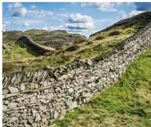
FIGURE 2.a.58 Fell top wall constructed from volcanic slate, Lingmoor, Langdale
