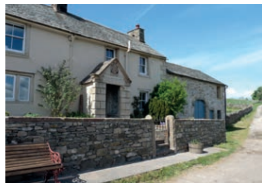
NO. 8 Widewath Farm
