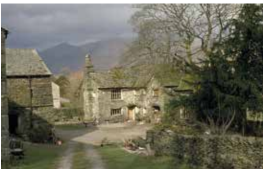
FIGURE 2.12 Statesman period farm at Low Fold, Troutbeck, displaying cylindrical chimney stacks, wooden window mullions and graded slate roof
