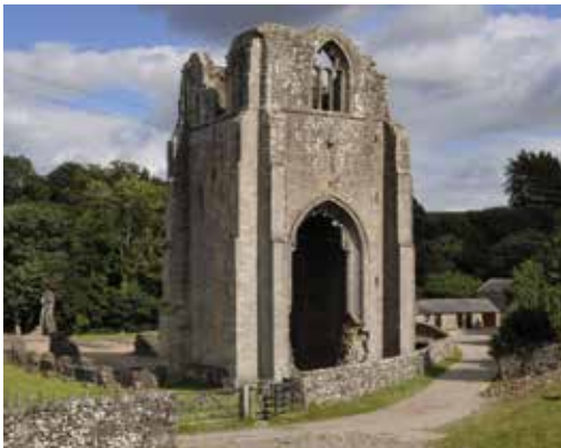
FIGURE 12.10 The remains of the tower and church at Shap Abbey
