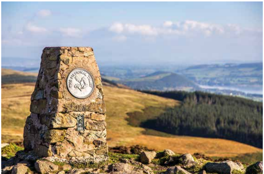
FIGURE 11.17 The Ordnance Survey's triangulation pillar on the summit of Gowbarrow Fell, with plaque recording ownership by the National Trust
