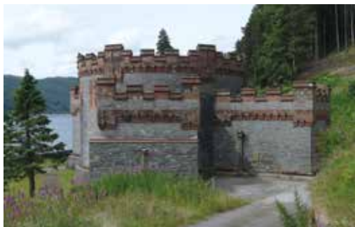
FIGURE 10.8 The Straining Well and Valve House for the Thirlmere Reservoir. Constructed 1885 – 1894 as a mock castle-like building intended to diminish its visual impact.
