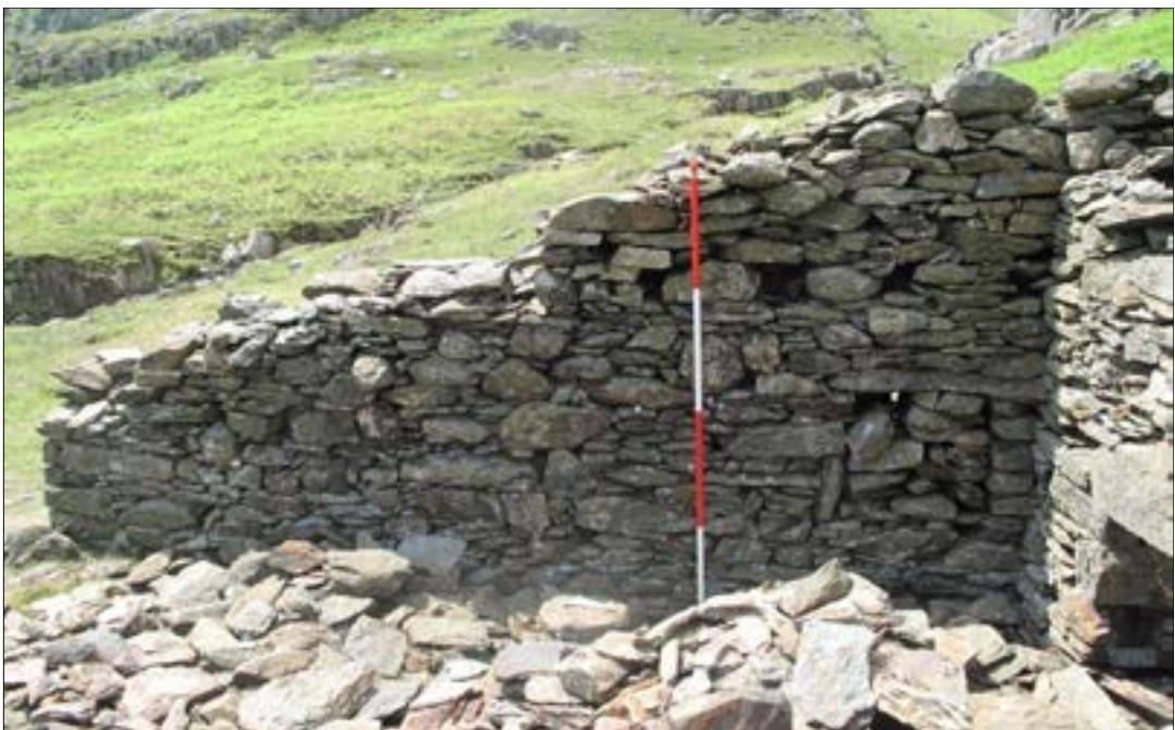
Plate 20: building 100; internal face of wall 110, showing timber slots above blocked window 111.
