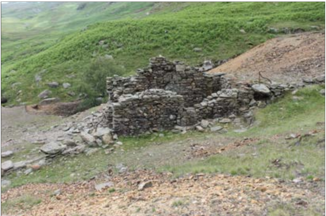
Plate 22: building 200 from the north.
