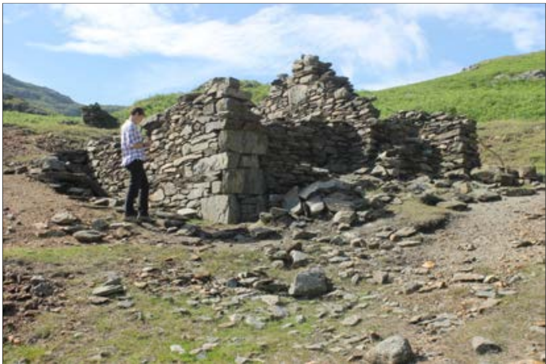
Plate 24: building 200 from the south-east. The figure is standing on the side of the wheel pit.
