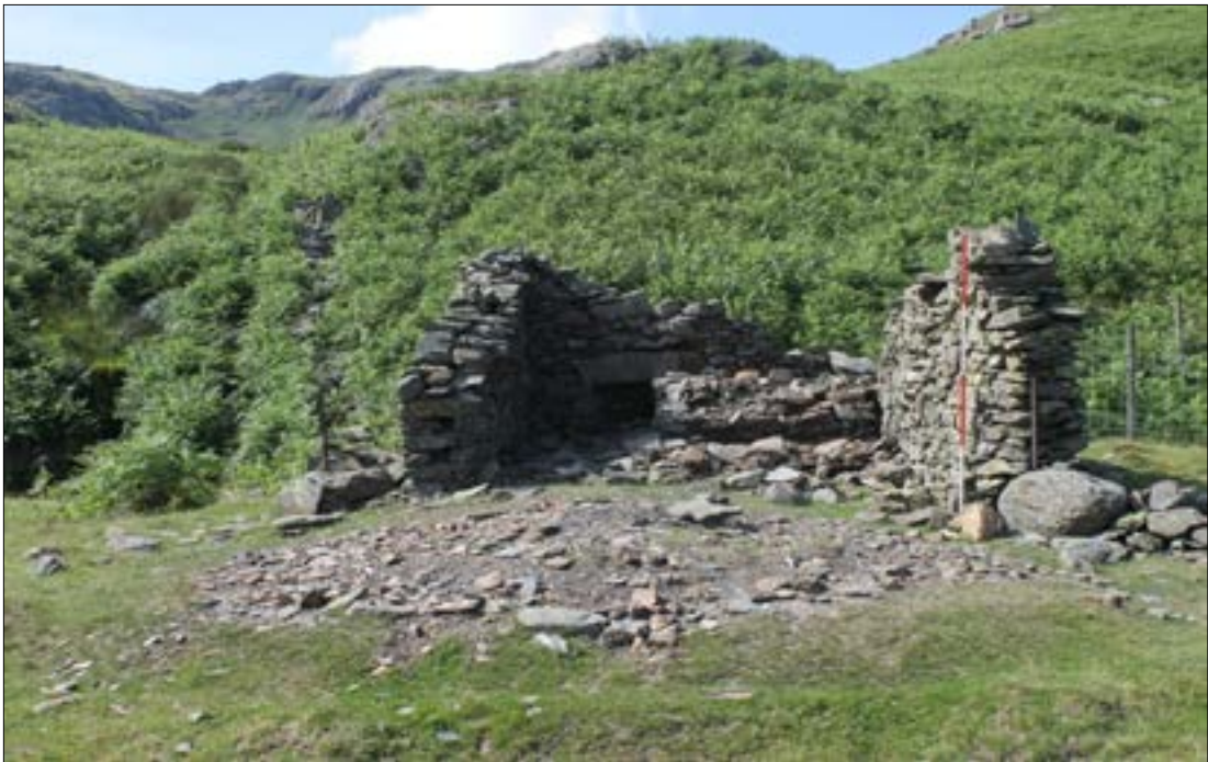
Plate 18: building 100 from the south showing hearth 121, with the plinth for the smithy hearth (140) in front.
