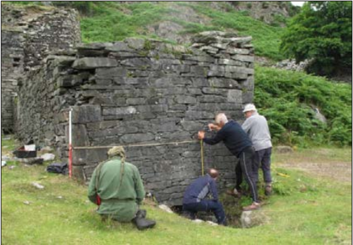
Plate 4: traditional building recording techniques – volunteers using tape and offset to record the east wall of the wheel pit
