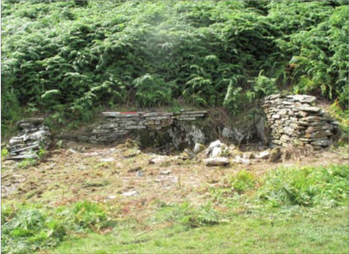
Plate 53: east-facing open-fronted riving shed (800)
