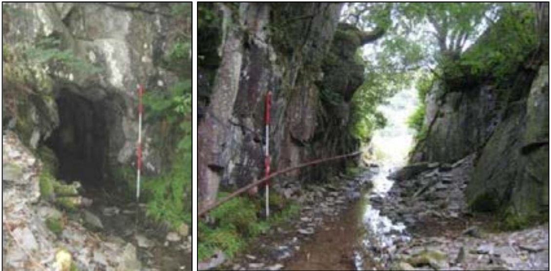
Plates 6, 7: (left) portal to Horse Crag Level (101) and (right) associated cutting (102), note water continues to drain out of the adit
