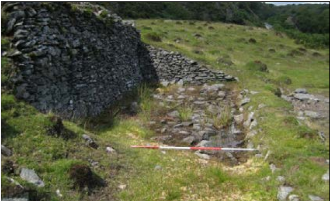
Plate 40: western settling pond (520), one of two to the north of the dressing mill. Water still pools in the base of the feature
