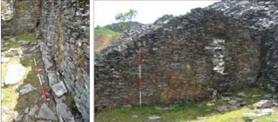
Plates 37, 38: (left) stone plinth (503) for carrying the launder channelling water to the settling ponds, and (right) north-facing elevation of south wall (507)
