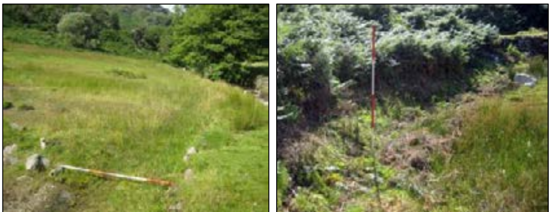
Plates 46, 47: (left) gap (607) at east end of bank (604), possibly associated with a sluice or overflow, and (right) low, discontinuous retaining wall forming curved S-section of tailings pond (602)
