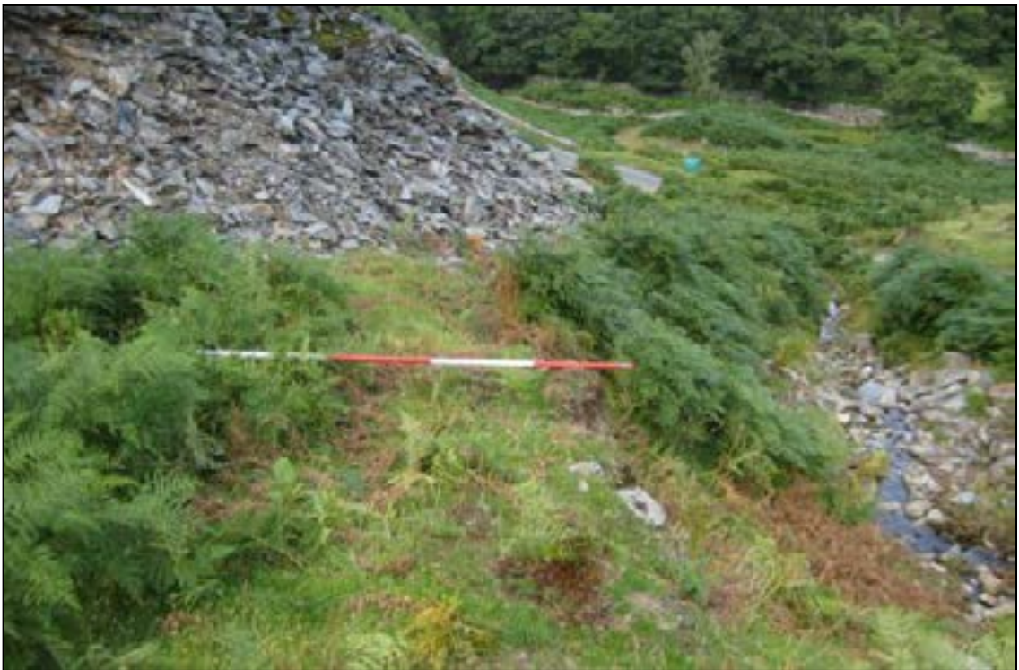
Plate 51: mine track (701), now overgrown and partially covered by waste from later quarrying
