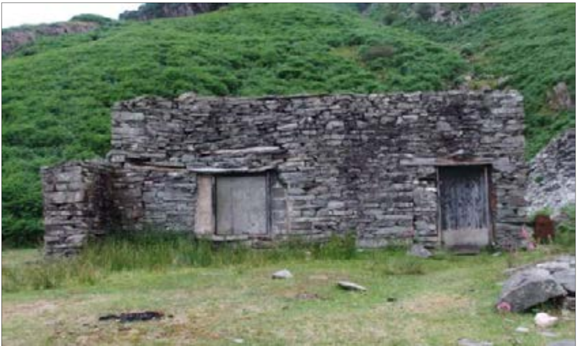
Plate 54: north-east-facing elevation (front) of riving shed (812)
