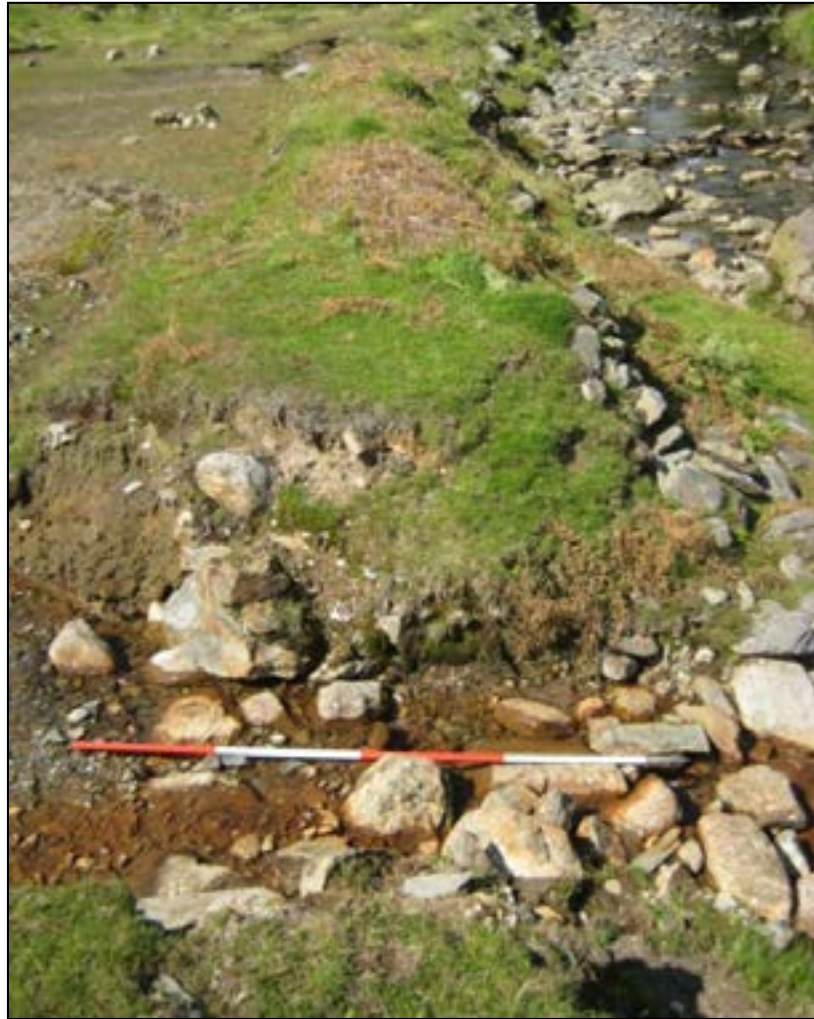
Plate 45: earth bank or levée (601) separating the tailing pond from Yewdale Beck
