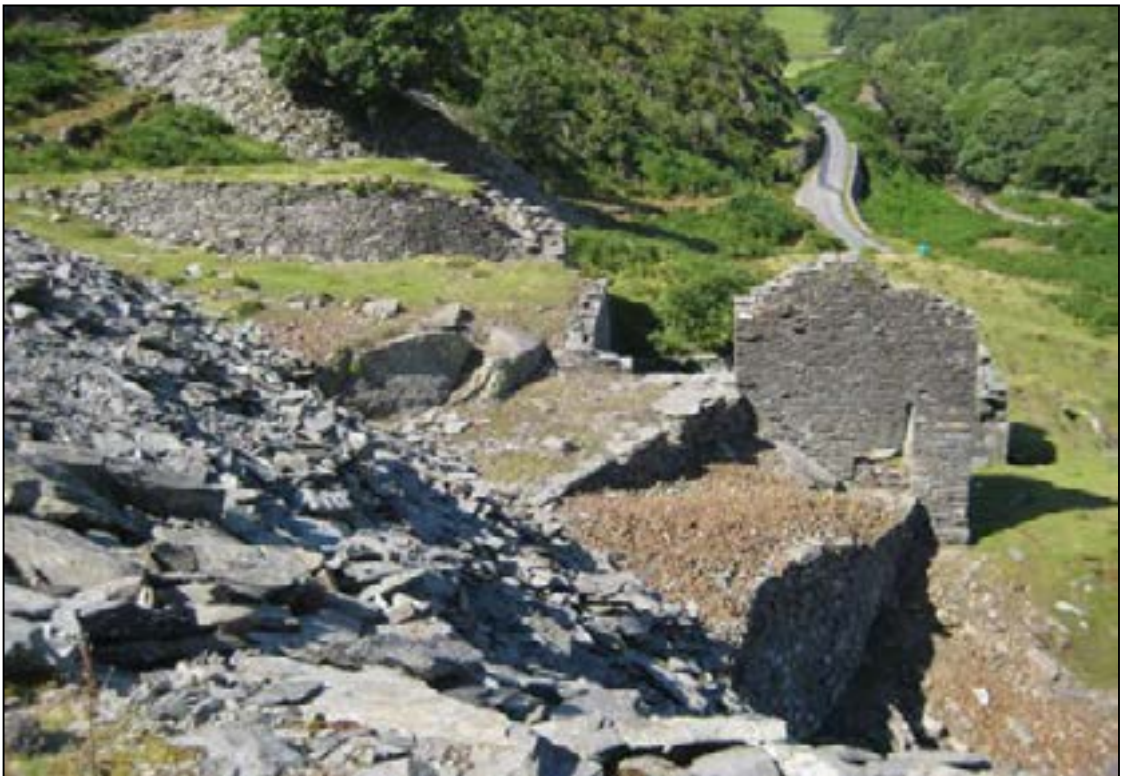
Plate 32: view of the southern gable of the crusher house showing the rectangular opening (410) and associated track way (414). The three retaining walls (417/418) and (415) are also visible
