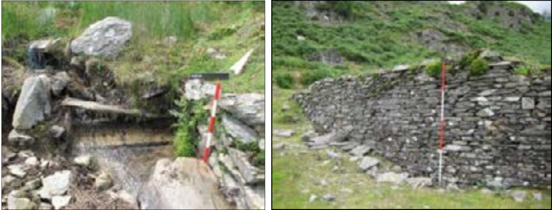
Plates 25, 26: (left) box-drain in leat (318) and (right) south wall of the holding pond (313); note collapse of east wall just visible on the left side of photo
