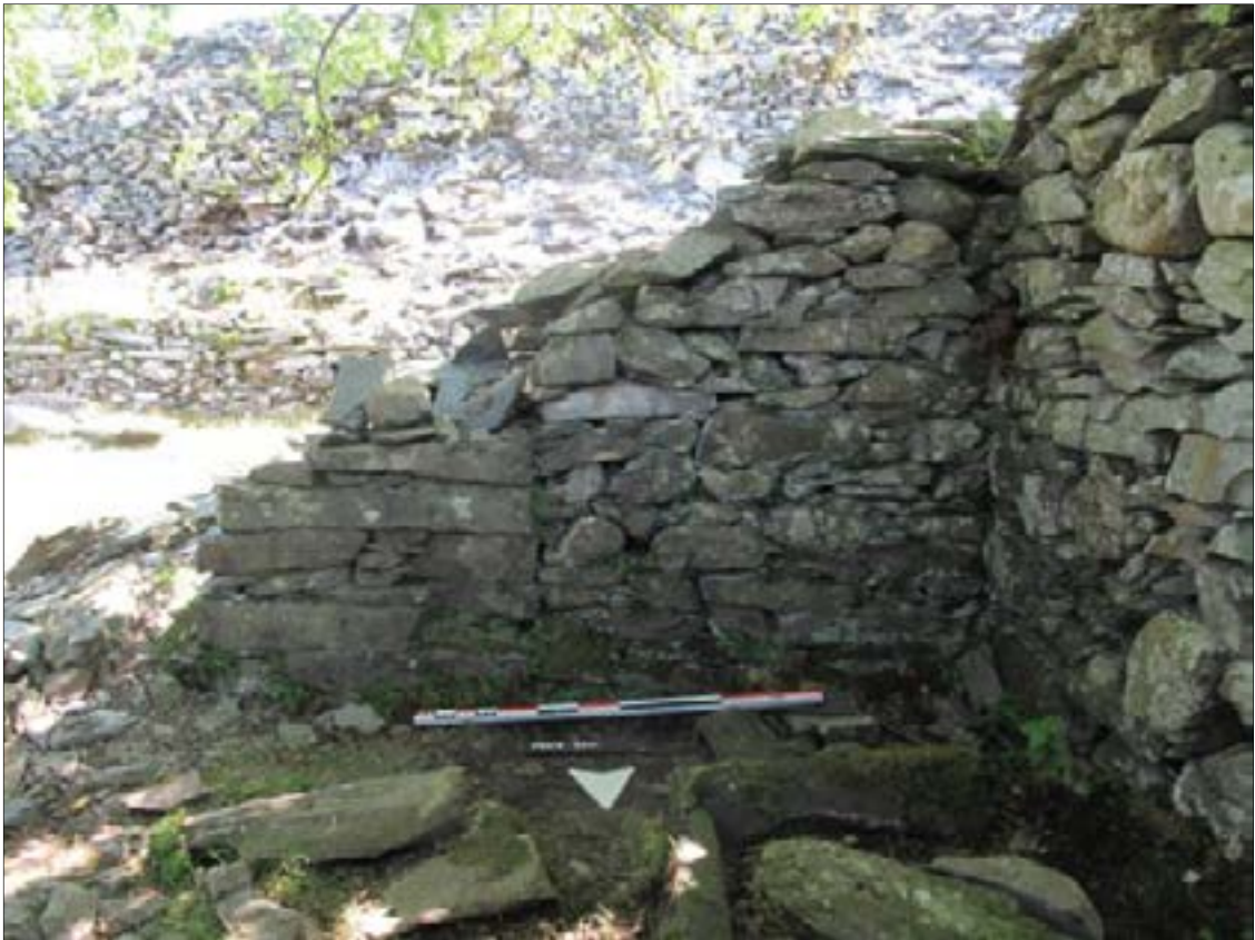
Plate 10: internal north elevation of wall (202), showing blocked door (203) to the left
