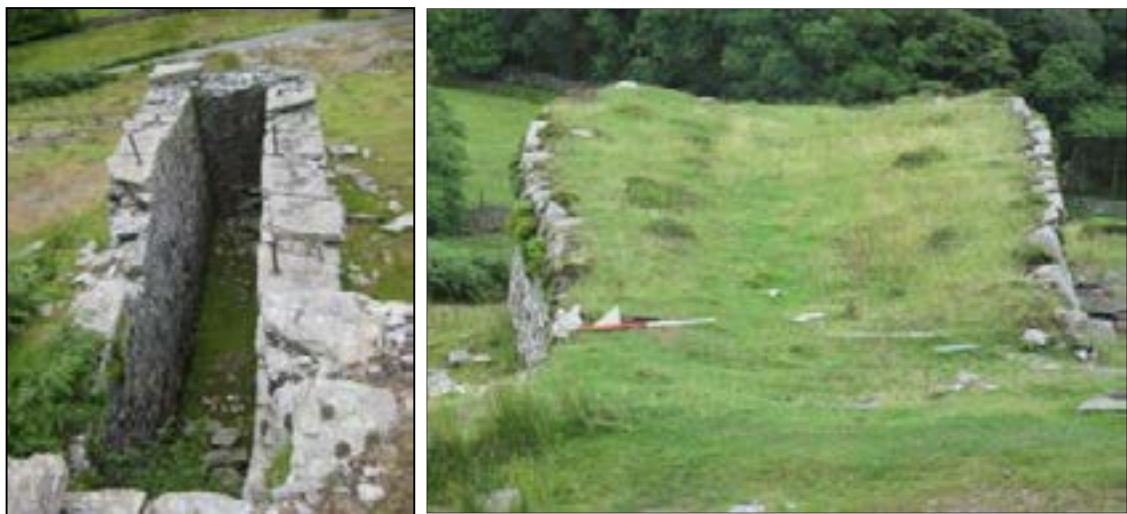
Plates 27, 28: (left) remains of the Penny Rigg wheel pit, with bolts for the horizontal wheel supports still in situ, and (right) turfed-over remains of the holding pond (310)
