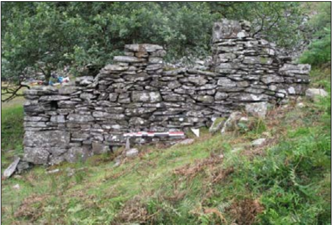
Plate 18: north-facing gable wall of smithy (201), looking south
