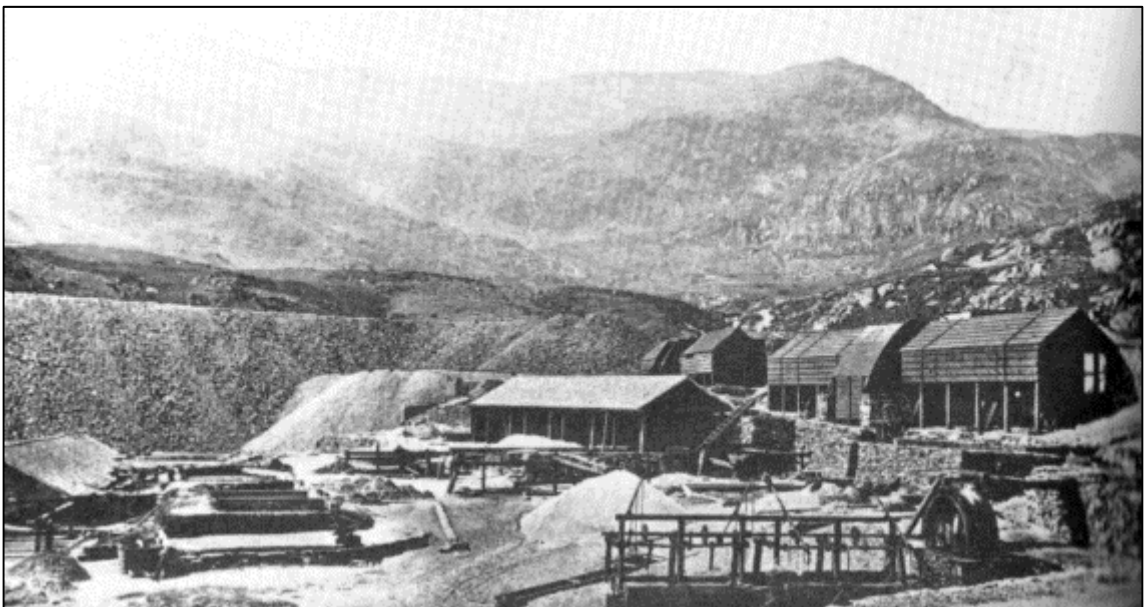
Plate 5: a late 19th-century view of the Bonsor Lower Mill at Coniston copper mines showing the extensive use of timber in the mill buildings. In the foreground is a set of unenclosed water powered jigs and to the left are open settling ponds. Taken from Holland 1986, 174
