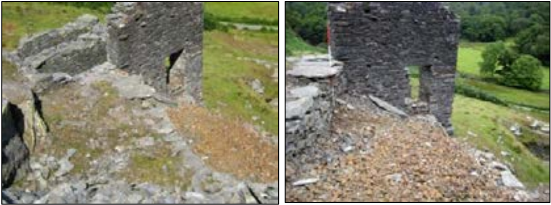
Plates 33, 34: tracks above the crusher for delivering ore: (left) upper track (416) delivering material via opening (409) and (right) the lower track (414) associated with the lower level opening (410)
