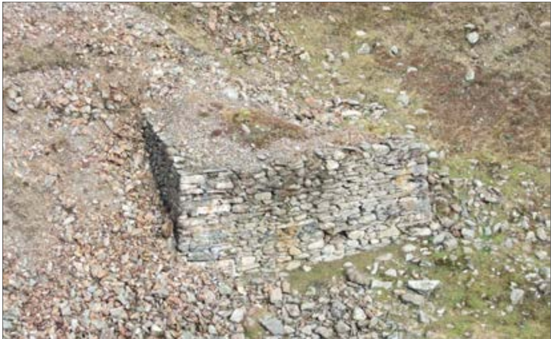
Plate 35: stone pier (340); the only surviving evidence of Stamping mill 1.
