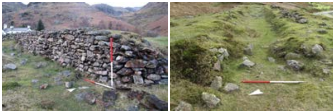
Plates 26 & 27: launder pillar associated with Stamping mill 3; retaining wall 213 (left) and grassed over top of feature (right).
