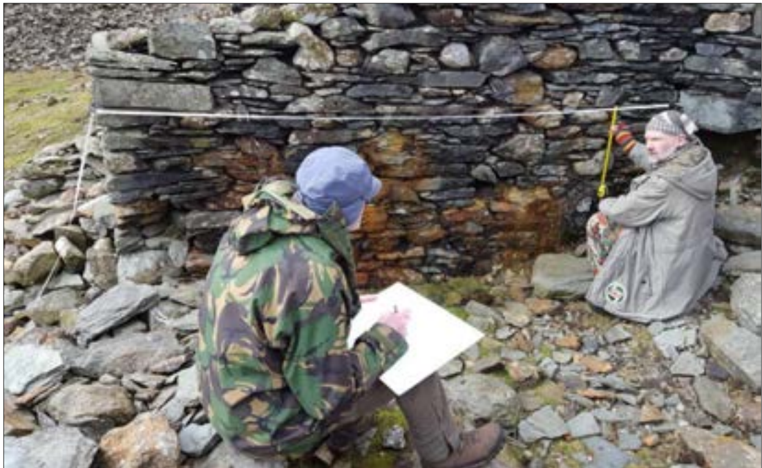
Plate 4: volunteers using tape and offset to record the office building (420).
