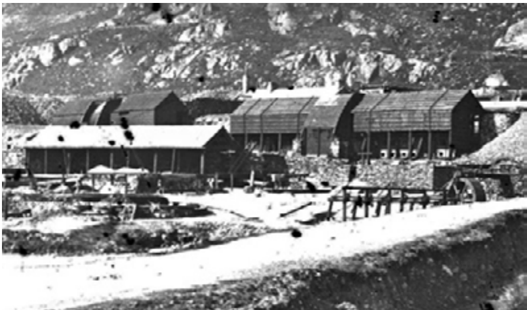
Plate 12: detail of P5 showing probable buddle sheds and stamp mill.
