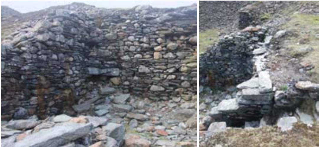
Plates 33 & 34: office west wall (424) and fireplace (423) (left) and view of structure looking west with steps (405) in the foreground.
