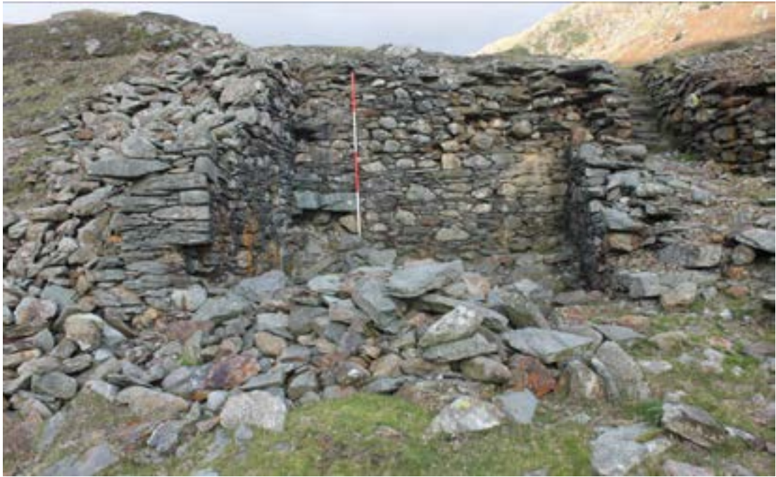
Plate 32: office building (420) looking north-west, steps visible to the left of the image.
