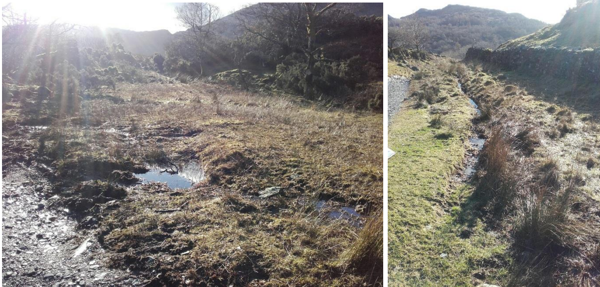
1 & 2: Looking down – old drains on right
