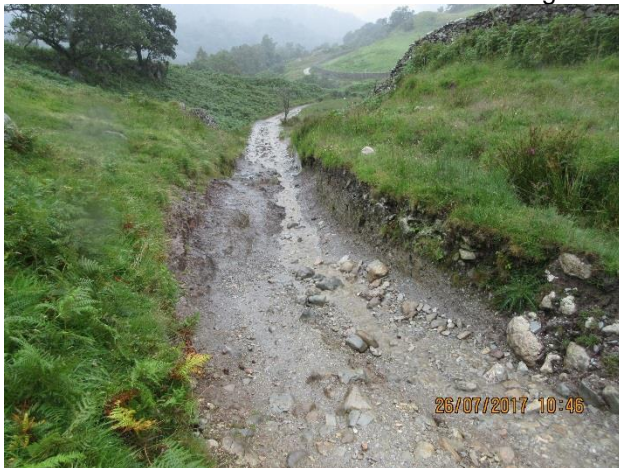
3: Looking down – old drains on right
