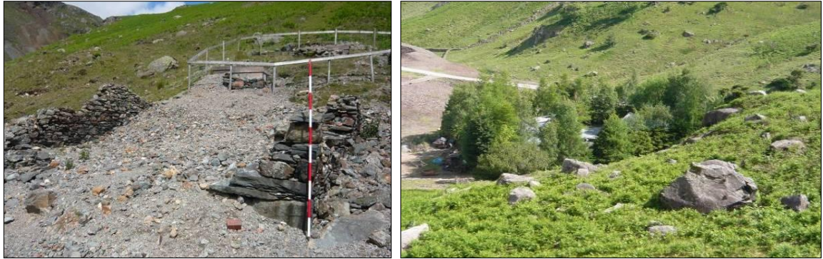
Plates 58 & 59: threats and issues. A burst water pipe associated with the Water Treatment Works virtually destroyed the offices at Paddy End and tree planting around the converted Old Powder Store is the subject of differences of opinion regarding their level of threat to the buried archaeology.
