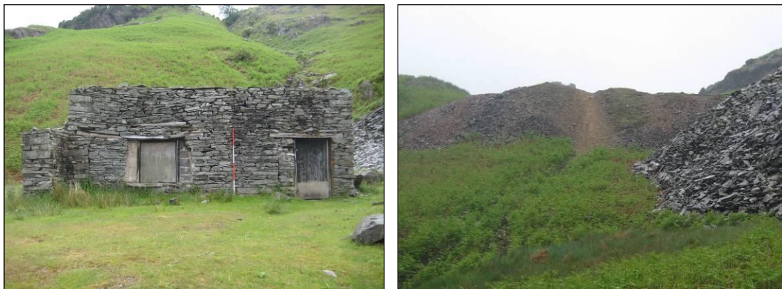
Plates 57 & 58: quarry building re-used as bothy (2032) note damage to window lintel and trail bike scars on the side of mineral waste tip (2055)
