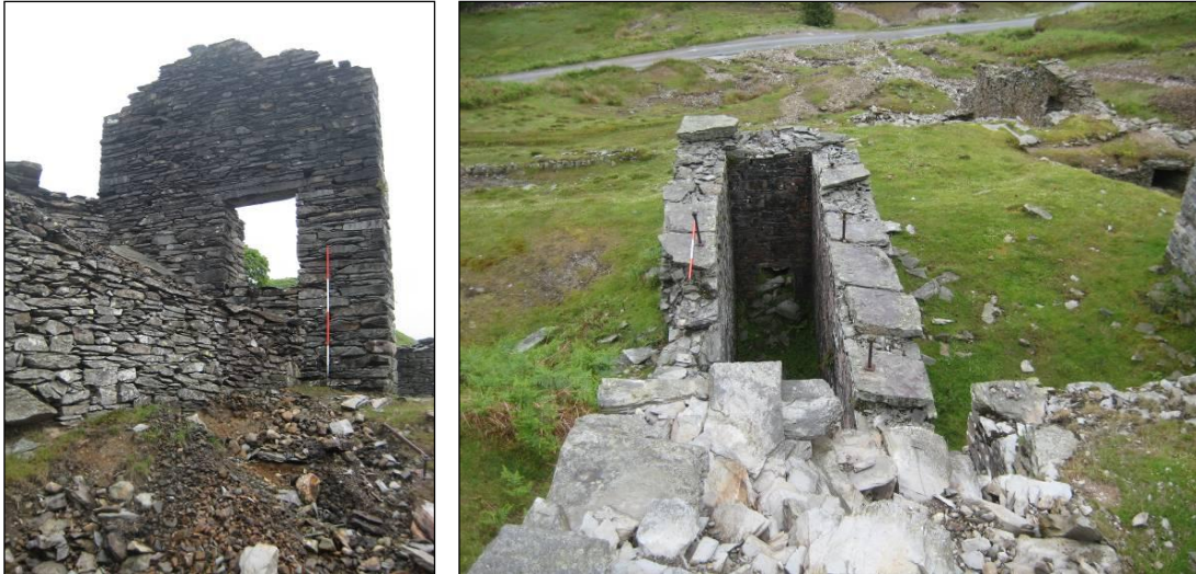
Plates 8 & 9: entrance to the upper floor of the crushing house still clearly preserved; ore was delivered via this directly to the upper floor of the crushing mill and then fed into the crusher below. And the wheel pit (2044) of the 32m diameter wheel which drove the crushing and stamping machinery – looking south from the holding pond (2045)
