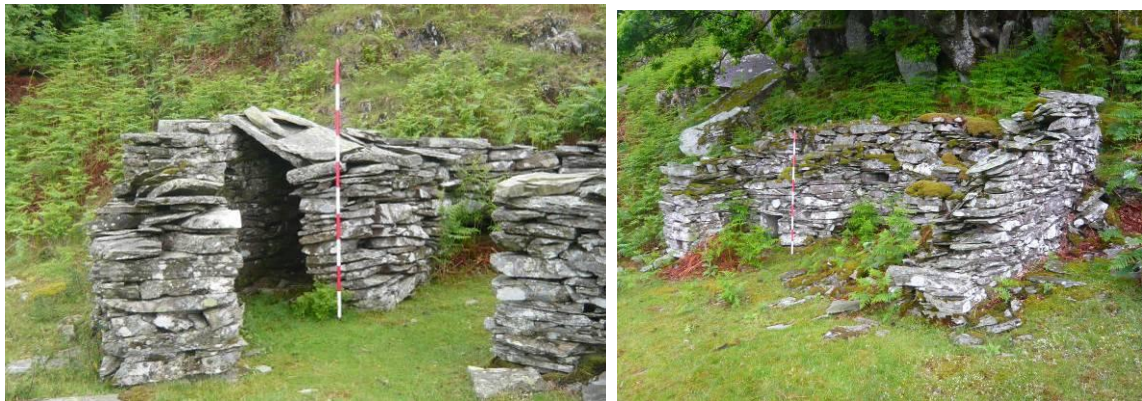
Plate 40 & 41: slate quarry buildings – the overall the preservation of these buildings is quite considerable, especially down the slope from the main Penny Rigg Quarry. These two buildings (2022) and (2031) lie on the south-east slope of Horse Crag. The first (2022) even has the slate slab roof preserved over the end cell.
