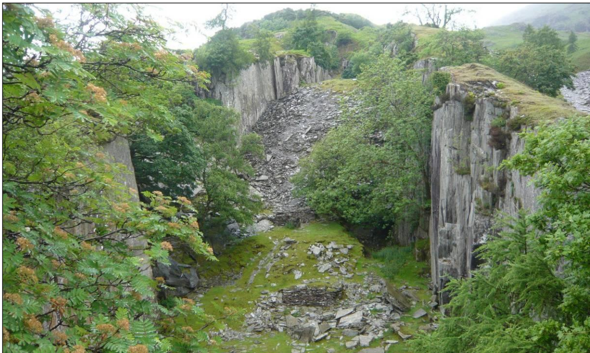
Plate 15: view south-west down Penny Rigg Quarry (2000) showing the progression of the terraces, with the older works at the lowest level in the foreground. The various structures at the base of the quarry are riving and processing sheds.
