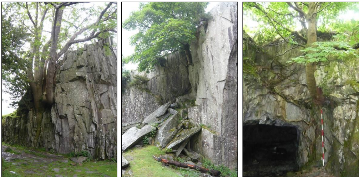
Plates 54 - 56: self seeded trees growing around Penny Rigg Quarry, the first in the wall of cutting (2013) the second on the north on the top terrace has caused a rock fall and the third above the closehead (2006) threatens to collapse the level entrance in the future.
