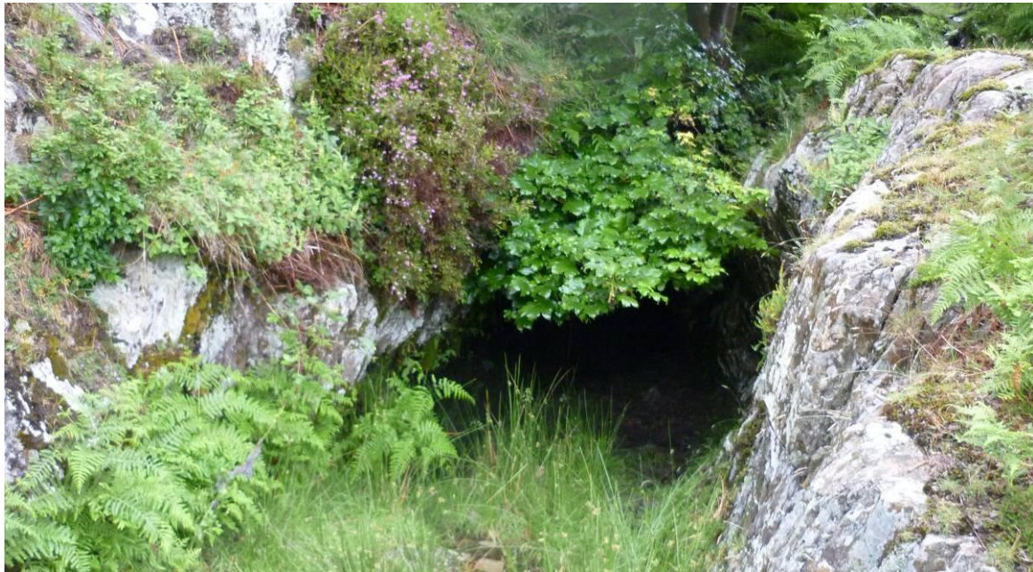
Plate 28: Entrance to mine on the south side of Penny Rigg quarry, excellent bat hibernation potential.
