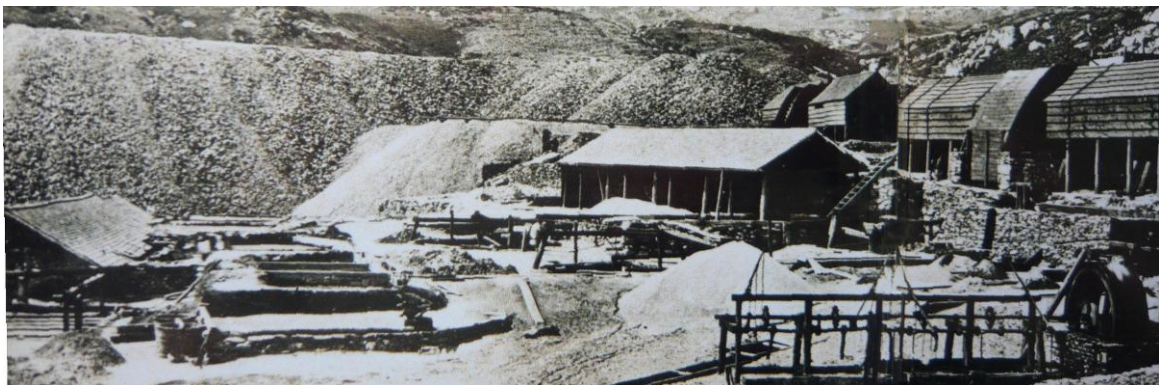
Plates 10: Dressing floors at Bonsor Low Mill at Coniston Copper Mine – a rack of jigs is clearly visible in the foreground and buddles to the left. The crushers were in the buildings to the right, on the terraces, while the large building in the middle may have been a bucking shed.
