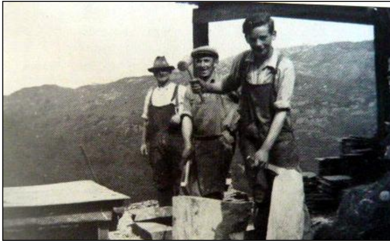
Plate 23: Splitting slate at Horse Crag Quarry - John W. Shaw in the background (from Holland 1986, 529)
