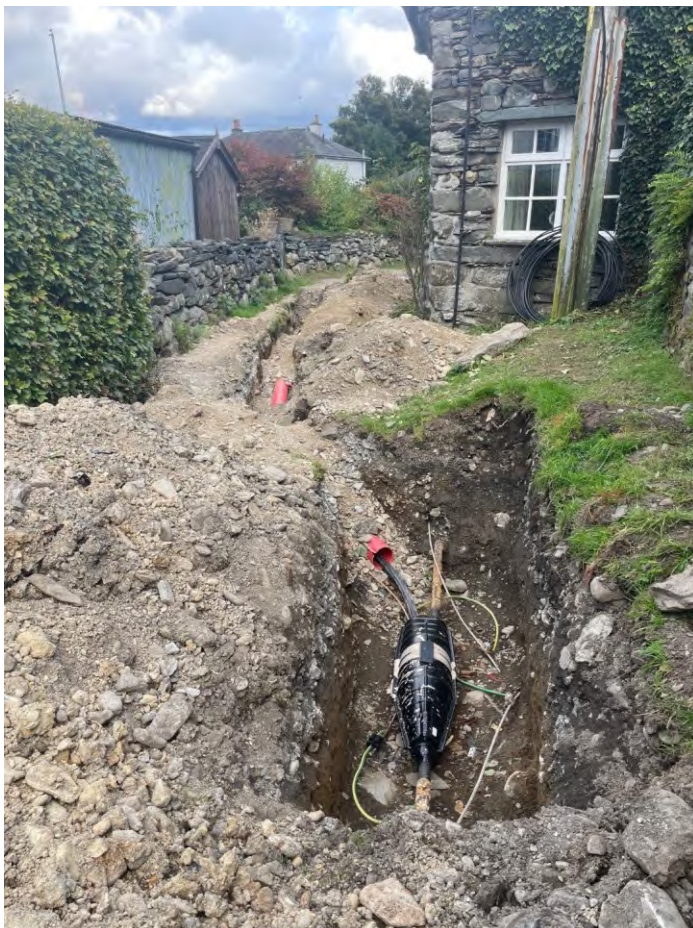
Path surface excavations
