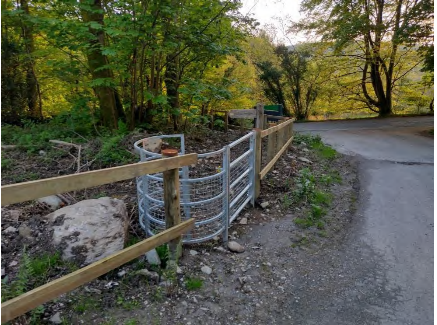
Annex 2 – Photo of kissing gate installed on Footpath 573029
