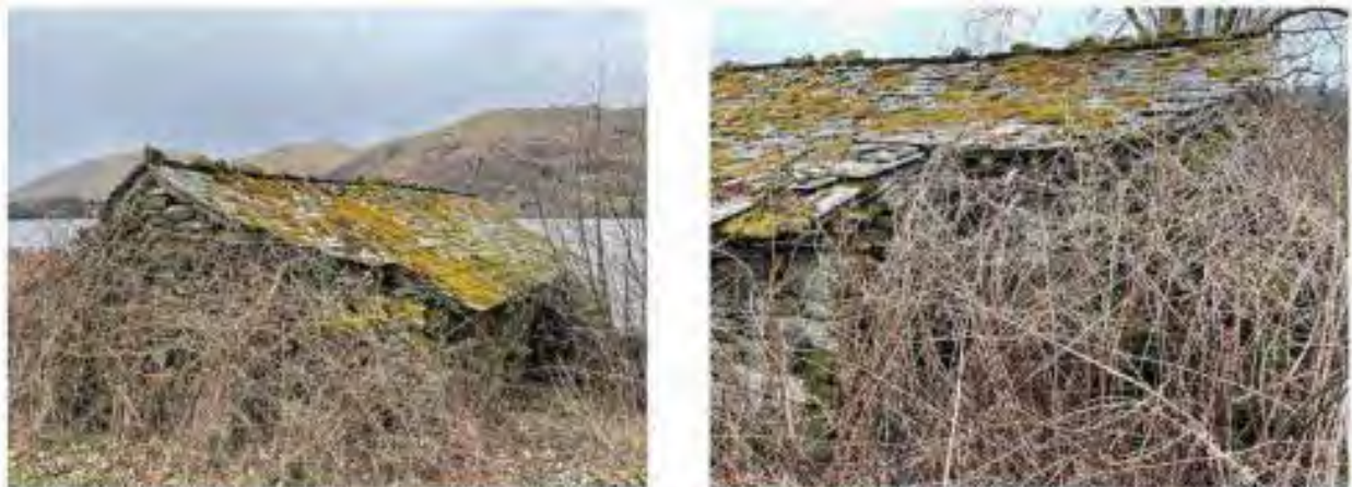
Photos of current condition of boathouse – taken from the bridleway.
