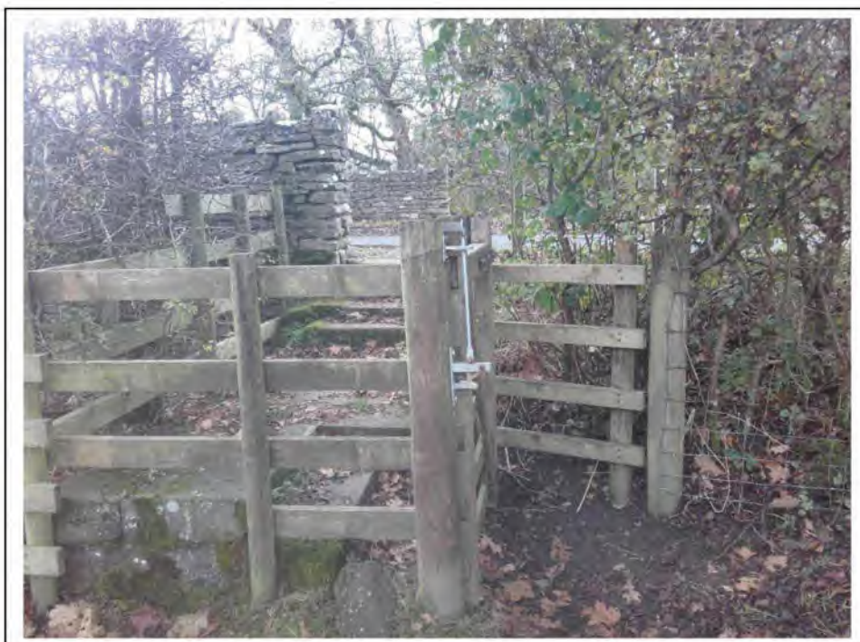
Photo 2: Point B, where extension of Millennium Path joins existing FP 306019 – steps to be replaced with pedestrian ramp
