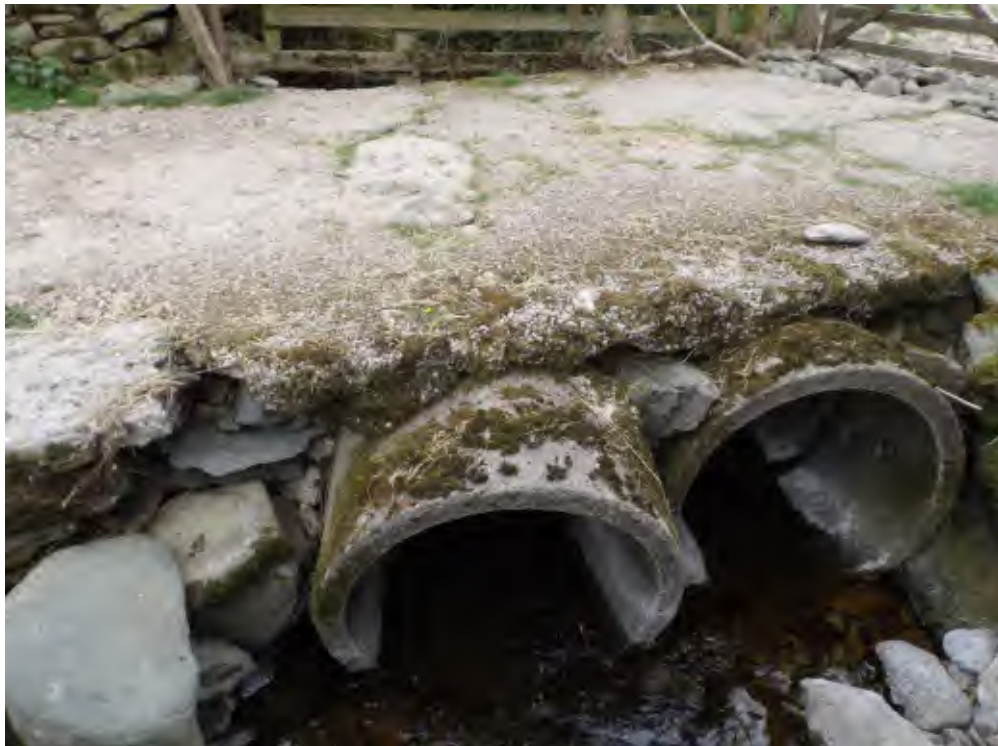
Figure 1: The existing culverted pipe crossing of Brown Beck
