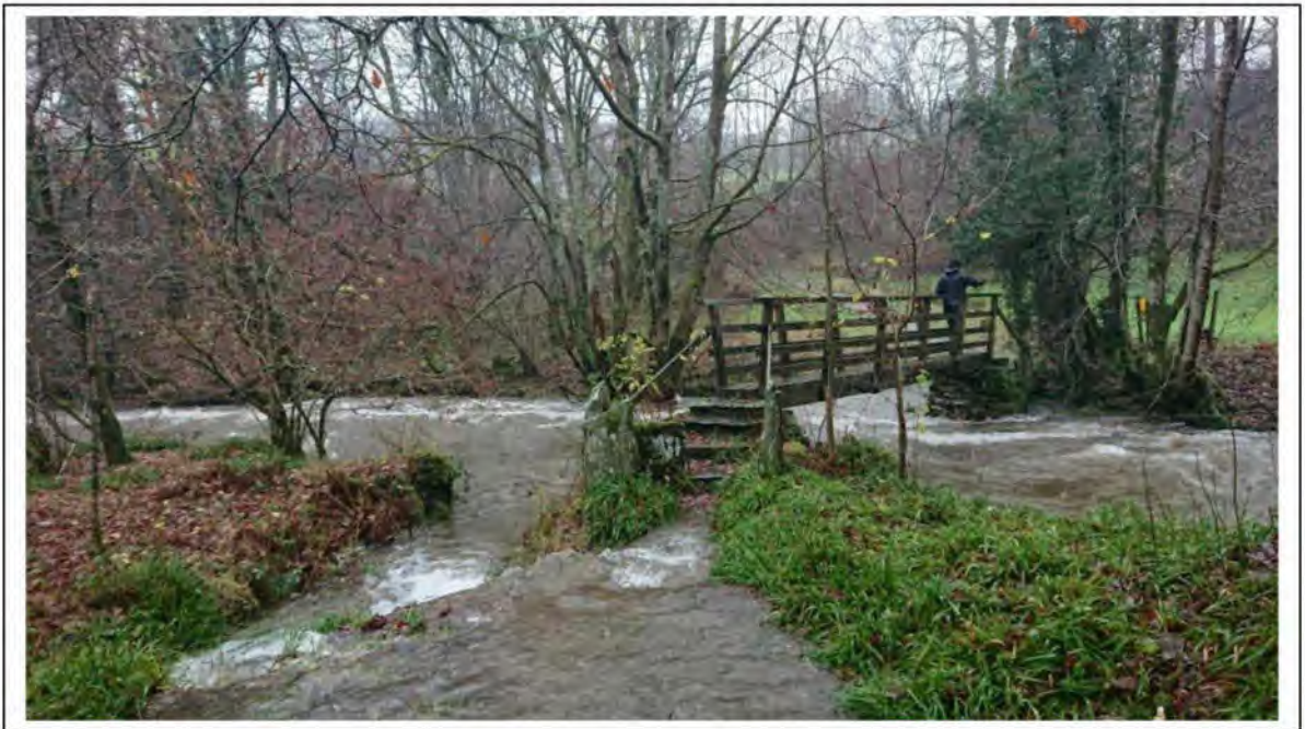
Photo 2: Bridge to be replaced
