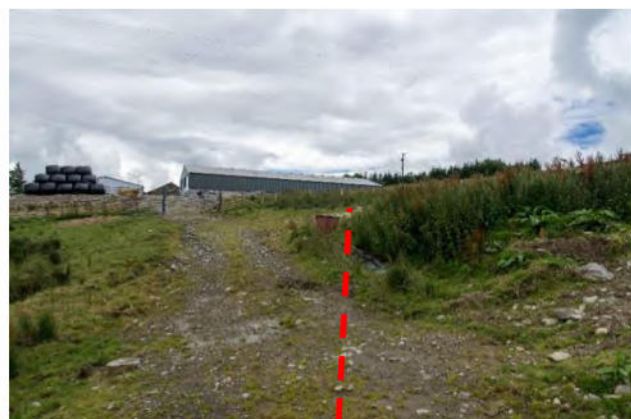
Looking south from Point C in 2015, along roughly the same line, after the barn and excavation work – this does not really show accurately the true depth of the excavation.
