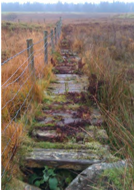
The short boardwalk between points F & H that will be replaced.
